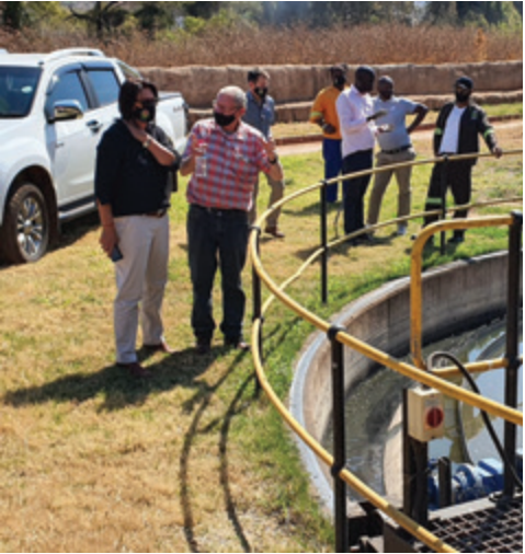
The PMT visited the Thabazimbi Wastewater Treatment Works.
